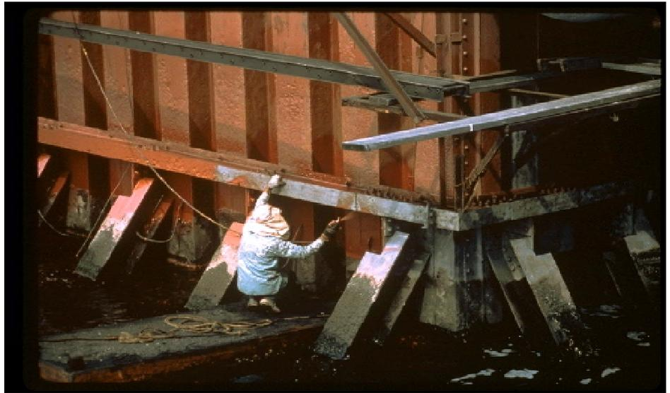
Airless spray equipment was used to apply Epodur®2755 urethane-modified epoxy primer to steelwork in the seaward corner of the coal-unloading pier. The corrosion-inhibitive primer is very tolerant of surface moisture, cures more quickly and at lower temperatures than conventional polyamide-epoxy primers, and provides excellent adhesion even in severely corrosive environments and in continuous immersion service.
